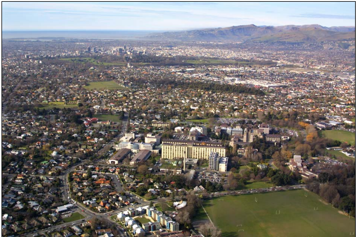
Figure 4: Photograph of Christchurch City
